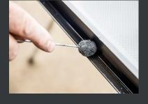
Degrease with beta wipe from kit round edge of cut hole and round edge of the frame turn frame over as its easy to do this way with lint free cloth in kit dry off shake little green top bottle for three mins and with the cotton bud from kit carefully prime 10mm wide round edge of hole and then round edge of frame let paint dry before moving on this takes around 5-10 minutes.
