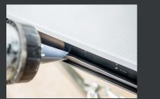
Remove backing foil from tube of glue in kit and pierce end with screw driver and then fit the pre cut nozzle from kit TIP HERE warm glue up before you start place on radiator or in bucket of hot water before you start with glue in gun you want a nice steady bead of glue all way round edge of frame there must be no gaps
