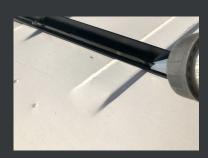
From the kit take a wipe from the kit and clean the frame and roof then with the primer and cotton bud supplied carefully prime round edge of the hole no more than 10mm or primer will show also prime frame face that meets the roof then leave five minutes to dry
